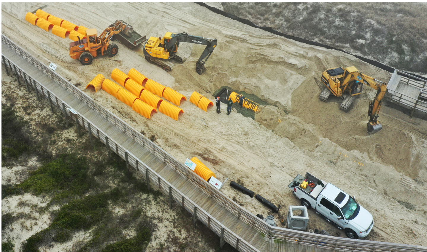
Dune Infiltration System (DIS), Caswell Beach, NC. Photo owned by WK Dickson.
