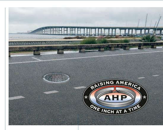
As the name implies, the AHP riser is a flexible, galvanized steel ring, with adjustability provided by a patented connecting turnbuckle. They're sized in 1/4" increments for thickness, starting at 3/4", so that new paving final grades can be matched precisely. The fully assembled risers can be ordered on short notice, but SWUCI keeps several on hand at all times, mostly in the 1" and 2" thicknesses that match local paving practice.
