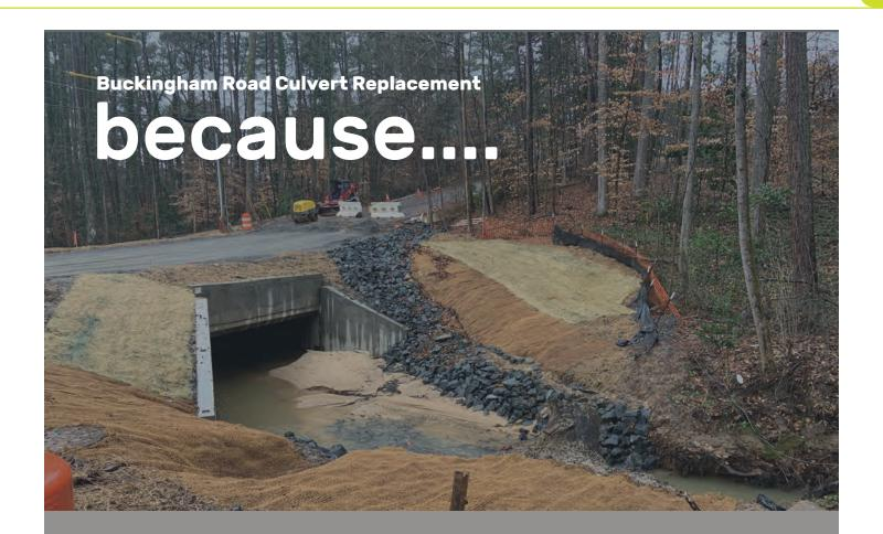
...the remnants of Hurricane Florence washed out a vulnerable, aging corrugated metal pipe culvert in a residential area of Durham, closing the road.
