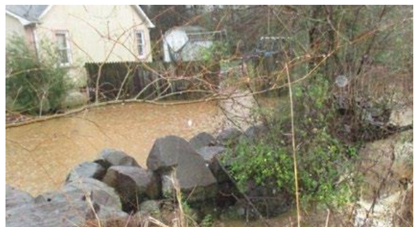
Flooding prior to flood mitigation project - September 2019 Newsletter
