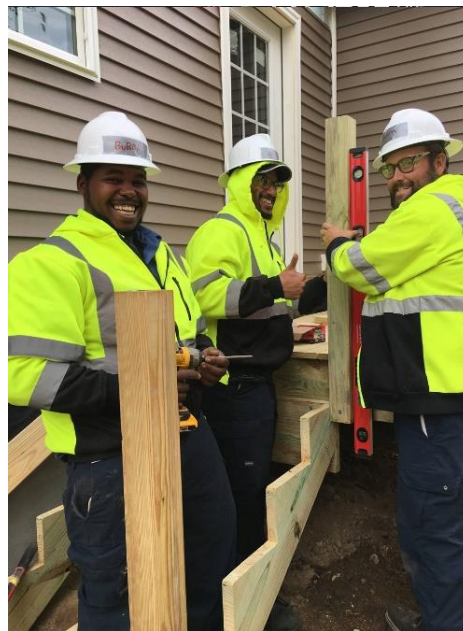
Habitat for Humanity Build
