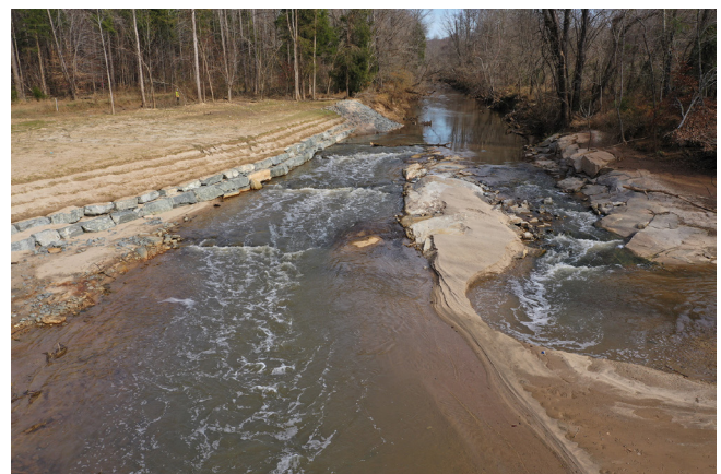
Salem Creek (after restoration)
